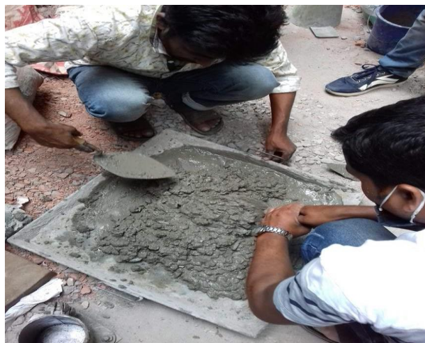
Figure No: 3.7 Mixing of Concrete
