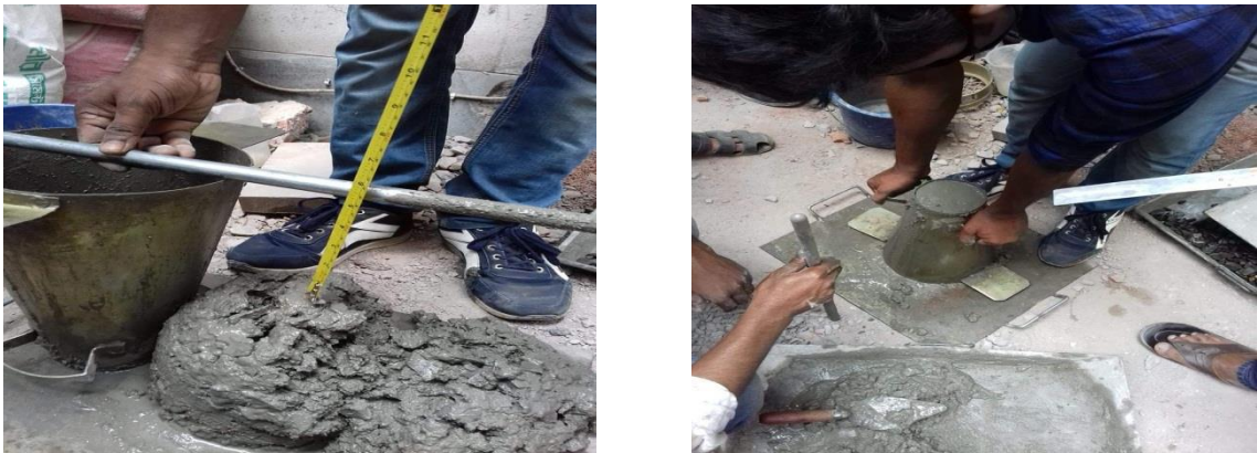
Figure No: 3.12 Slump Measurement
