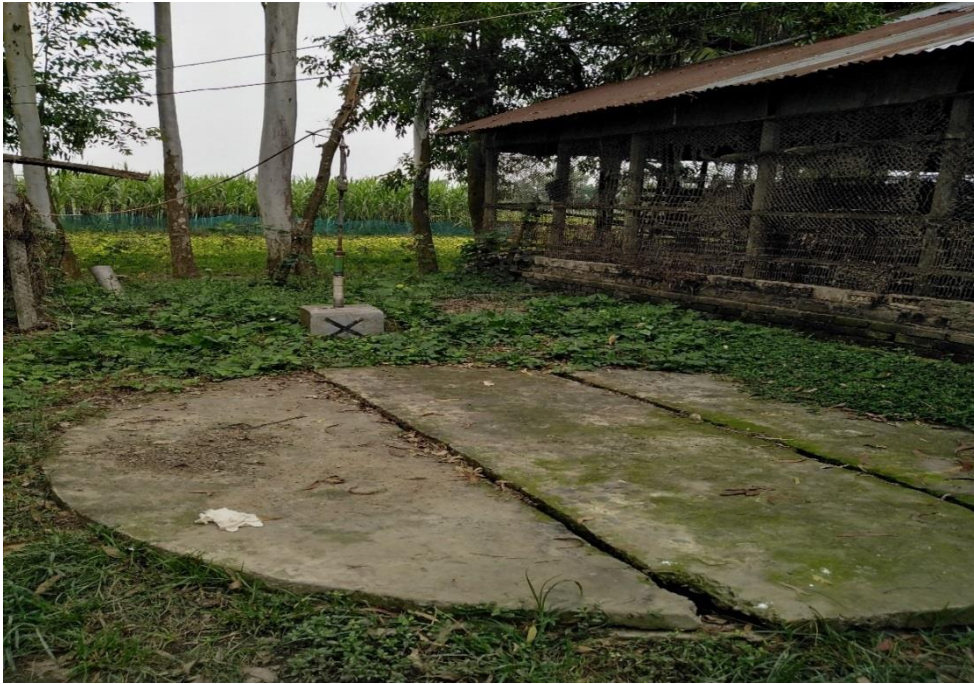
Fig.3.4: Bio gas plant
