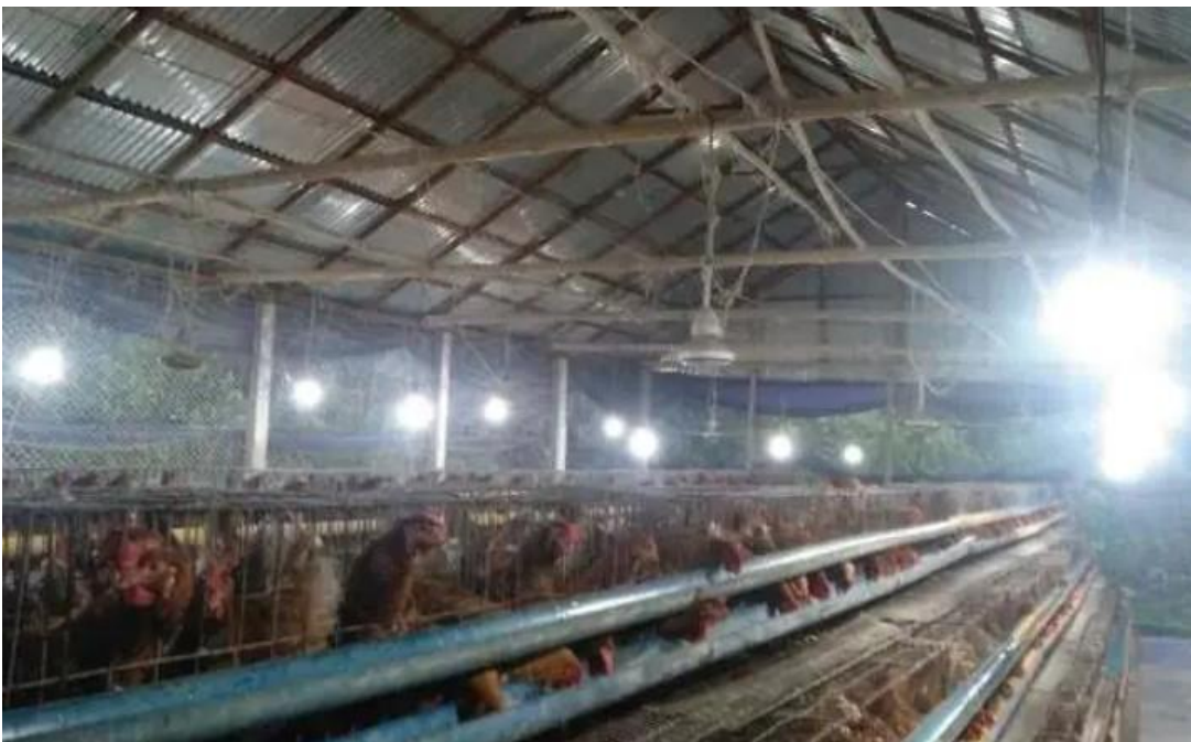
Fig.3.3: Layer farm lighting.
